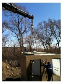
The green septic tape can be placed around the perimeter of the toilet body in preparation of the roof being set in place. The tape should be placed om the seam.
